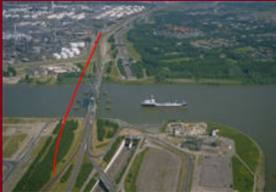
Botlek Railway tunnel
