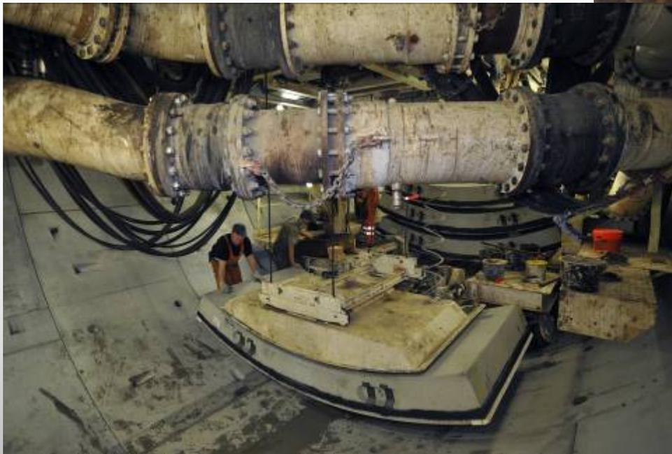
Longitudinal transport of a tubbing segment to the erecting device
