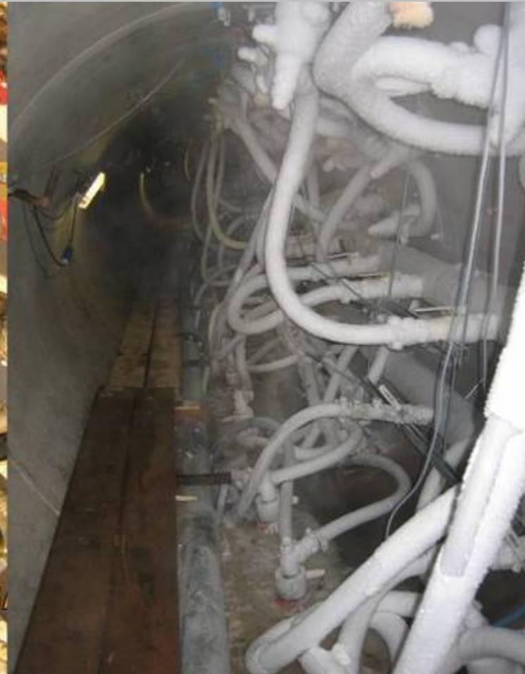
Soil freezing : freezing installation within the auxiliary gallery
