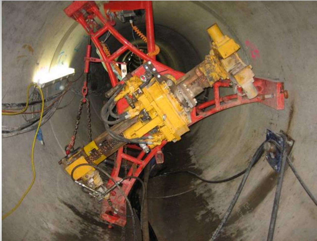
**Special drilling boom for freezing boreholes**
