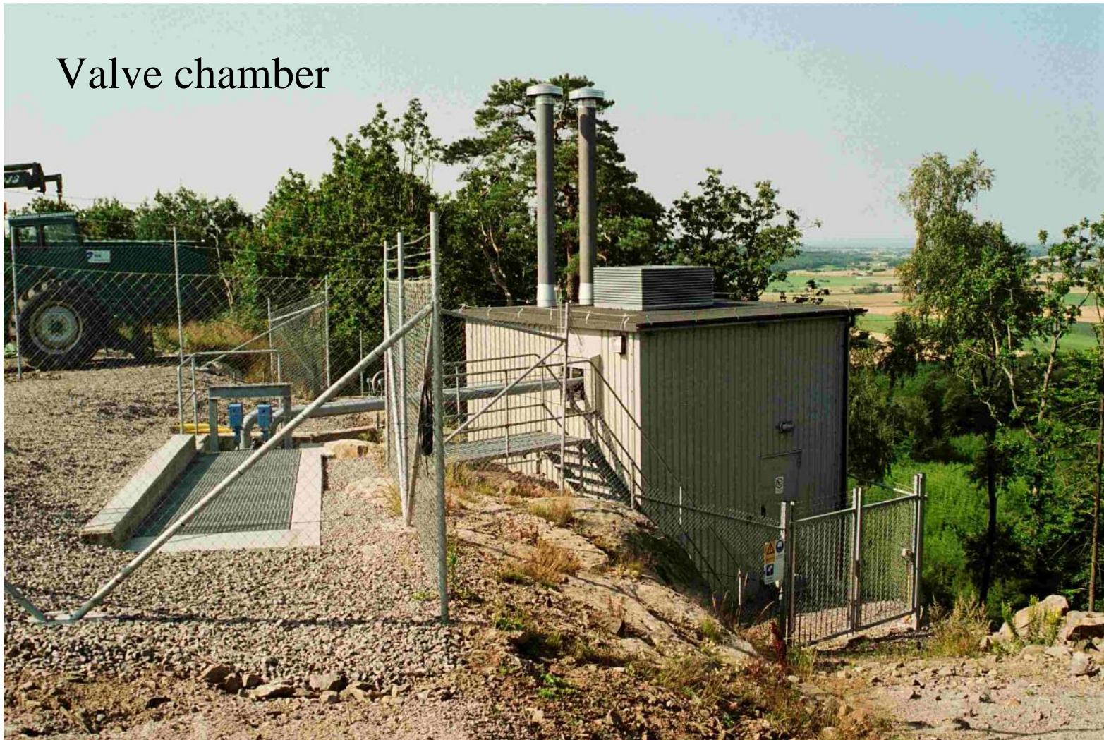
The valve chamber on top of the shaft houses the equipment at the well-head
