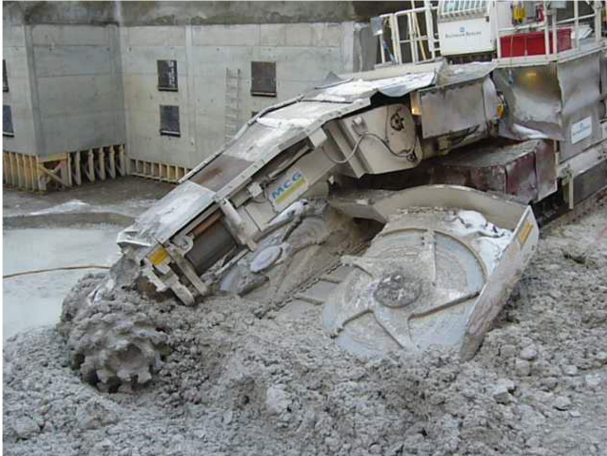
Bulk Excavation Roadheader
