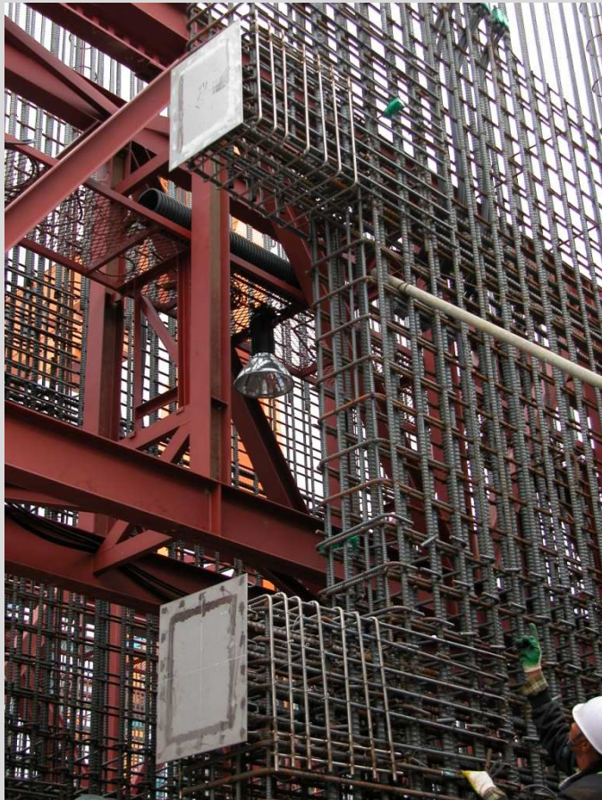
Rebars at shear keys
