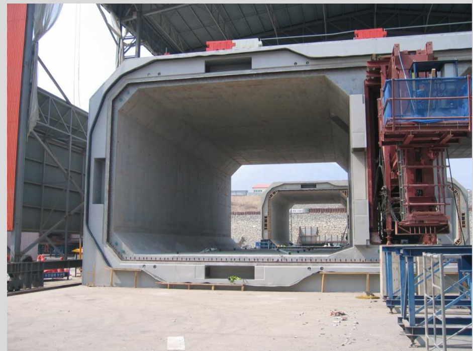
Example of segmental casting
