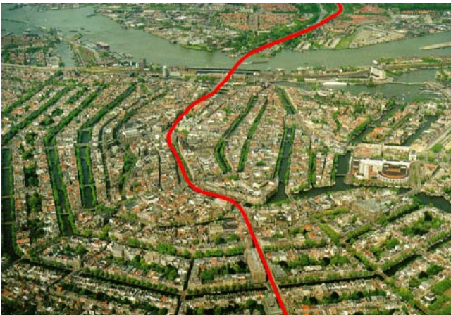
South Line Project
