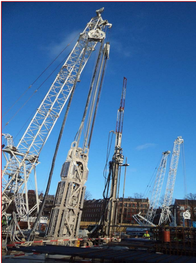
Figure. Diaphragm wall construction using hydro mill cutters.
